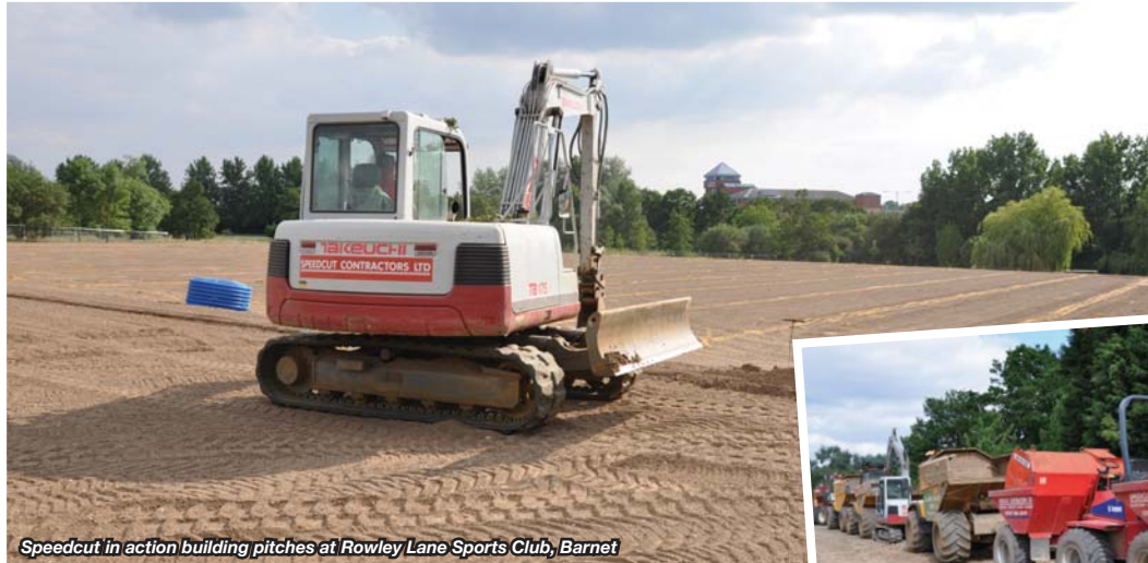
Speedcut in action building pitches at Rowley Lane Sports Club, Barnet
