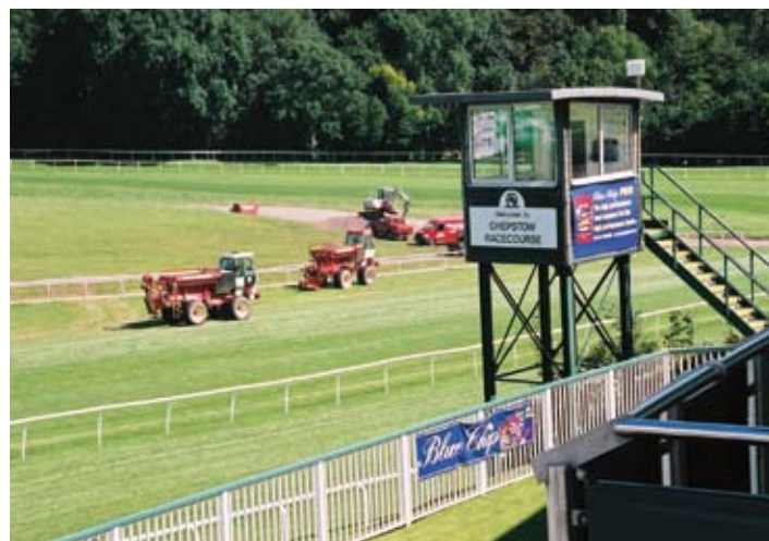
Speedcut Contractors at work on Chepstow Racecourse in August
